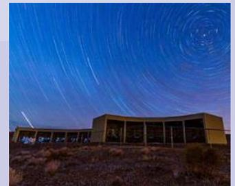
*This time-lapse photo shows the Middle Drum fluorescence detector station at the sprawling \$25 million Telescope Array cosmic ray observatory near Delta, Utah. The current observatory includes three such telescope stations, which contain mirrors to detect faint blue flashes in the sky when an incoming cosmic ray hits gas in the atmosphere.*
