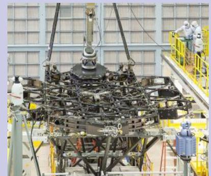
*The James Webb Space Telescope team successfully installed the first flight mirror onto the telescope structure at NASA's Goddard Space Flight Center in Greenbelt, Maryland. Credits: NASA/Chris Gunn*
