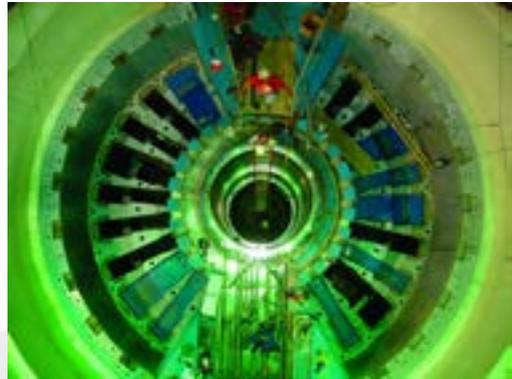
A massive part of Oak Ridge National Laboratory's Spallation Neutron Source is shown during its construction phase in earlier years. The hole in the center is where the target crystal for neutron scattering is placed. Credit: Oak Ridge National Laboratory
